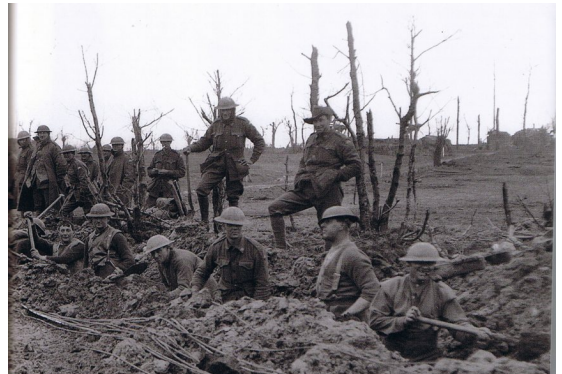
Right: Digging Trenches
